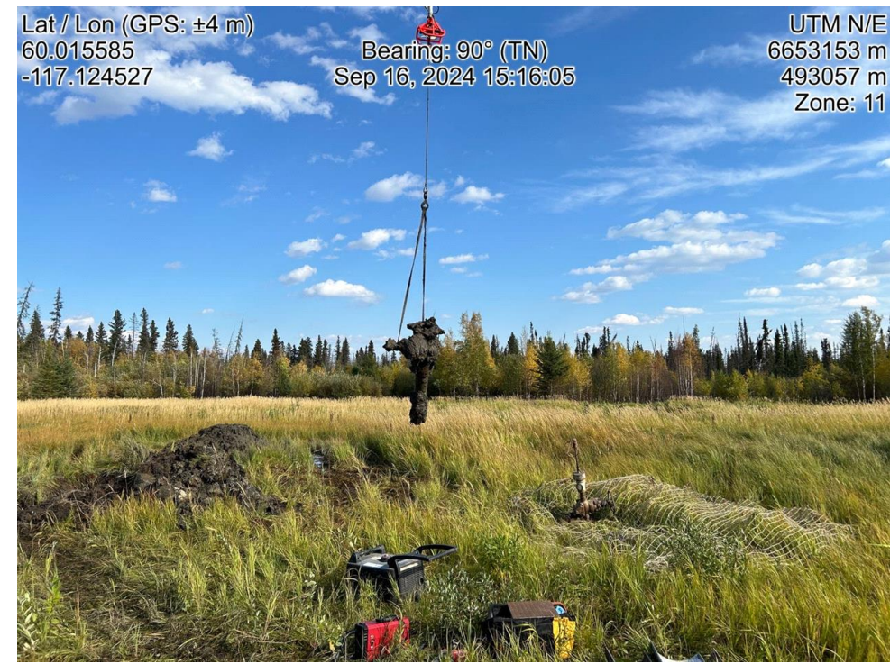
Wellhead removed with helicopter
