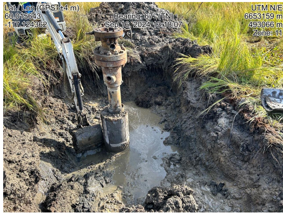
Excavating around wellhead
