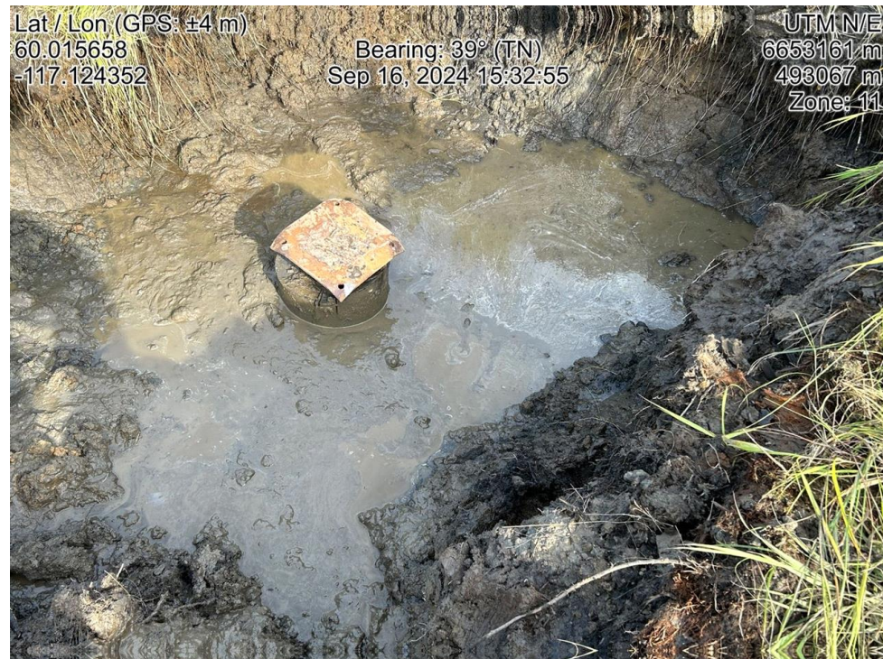
Vented cap welded onto casing stub
