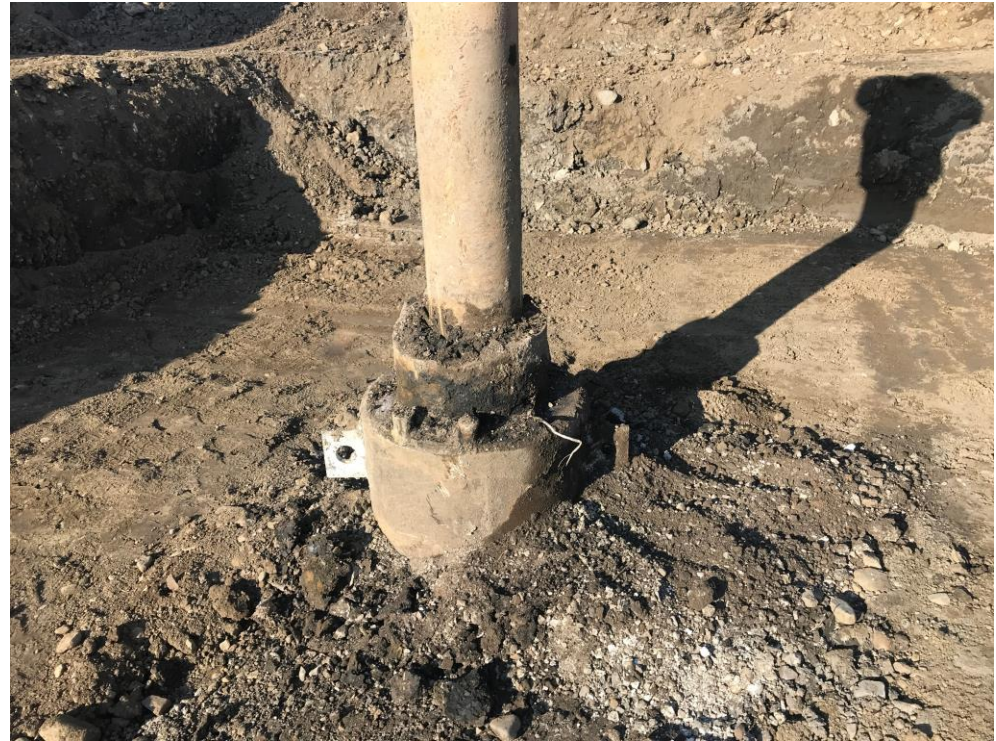
Wellhead and casing following excavation
