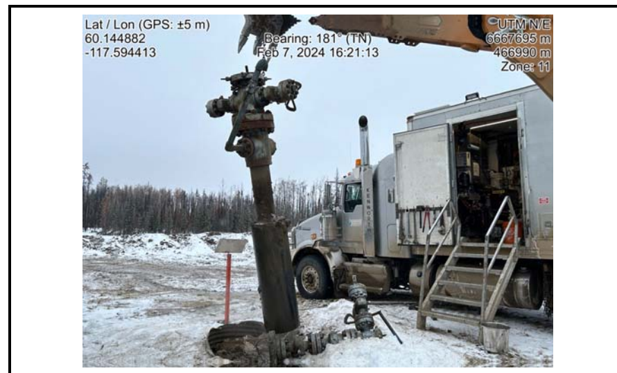
Wellhead cut and being removed
