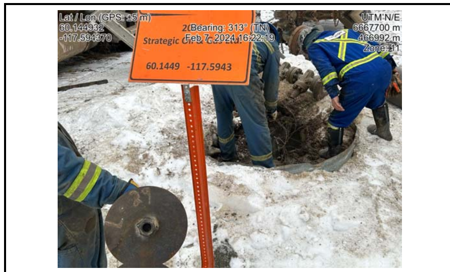
Crew inspecting the cut and the vented cap with "L-29" Welded in place
