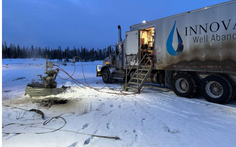
Wellhead taken apart and cutting tool installed
