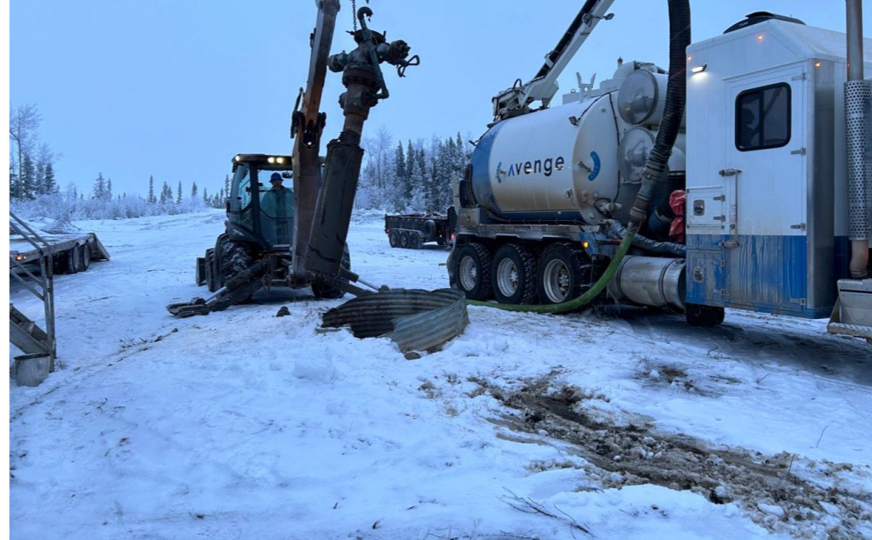
Wellhead cut and being removed
