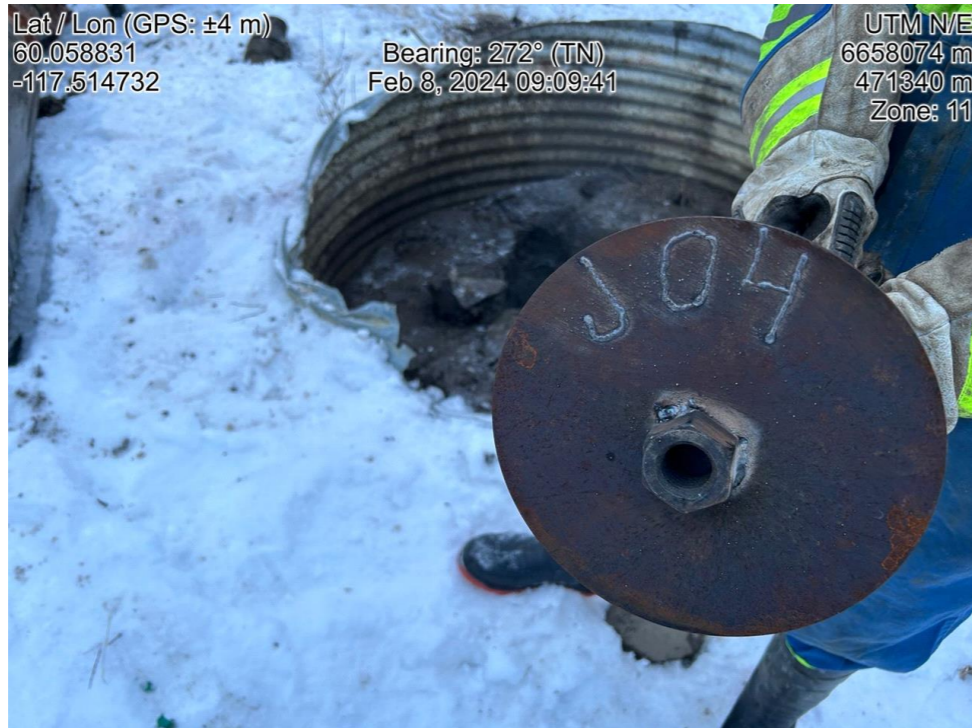
The vented cap with "J-04" Welded in place
