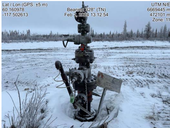
Wellhead with bubble test in progress.
