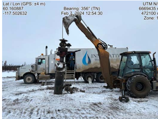
Wellhead cut and being removed
