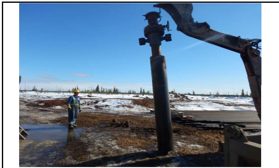
Wellhead pulled out of ground
