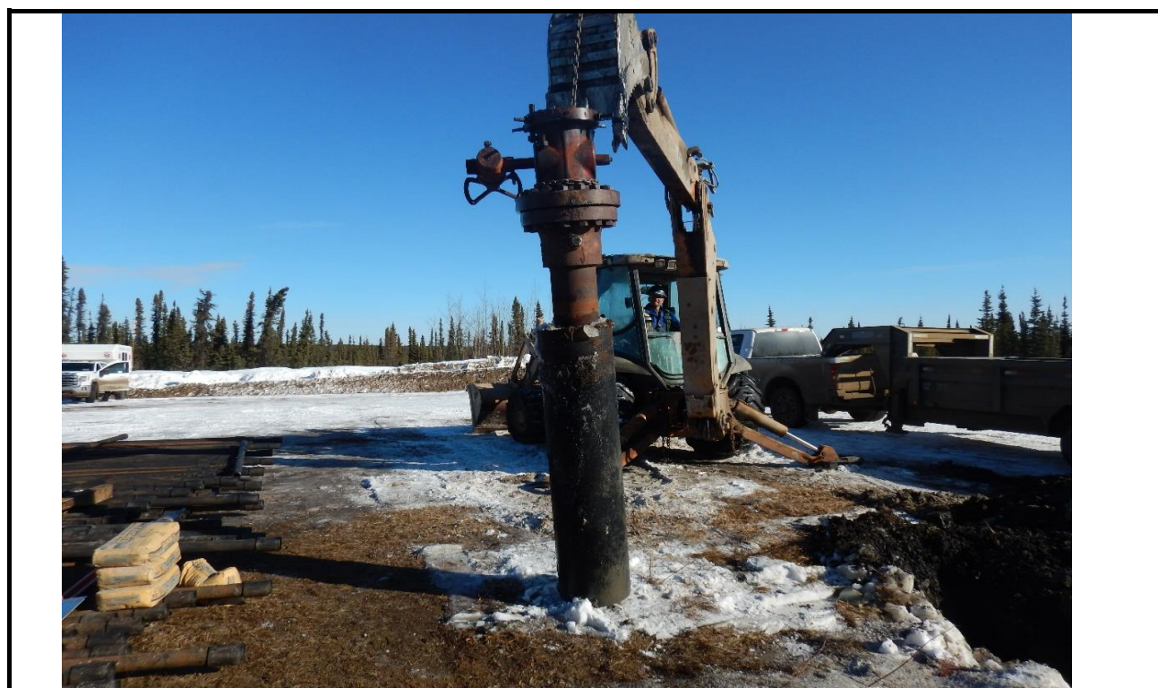
Wellhead removed from ground
