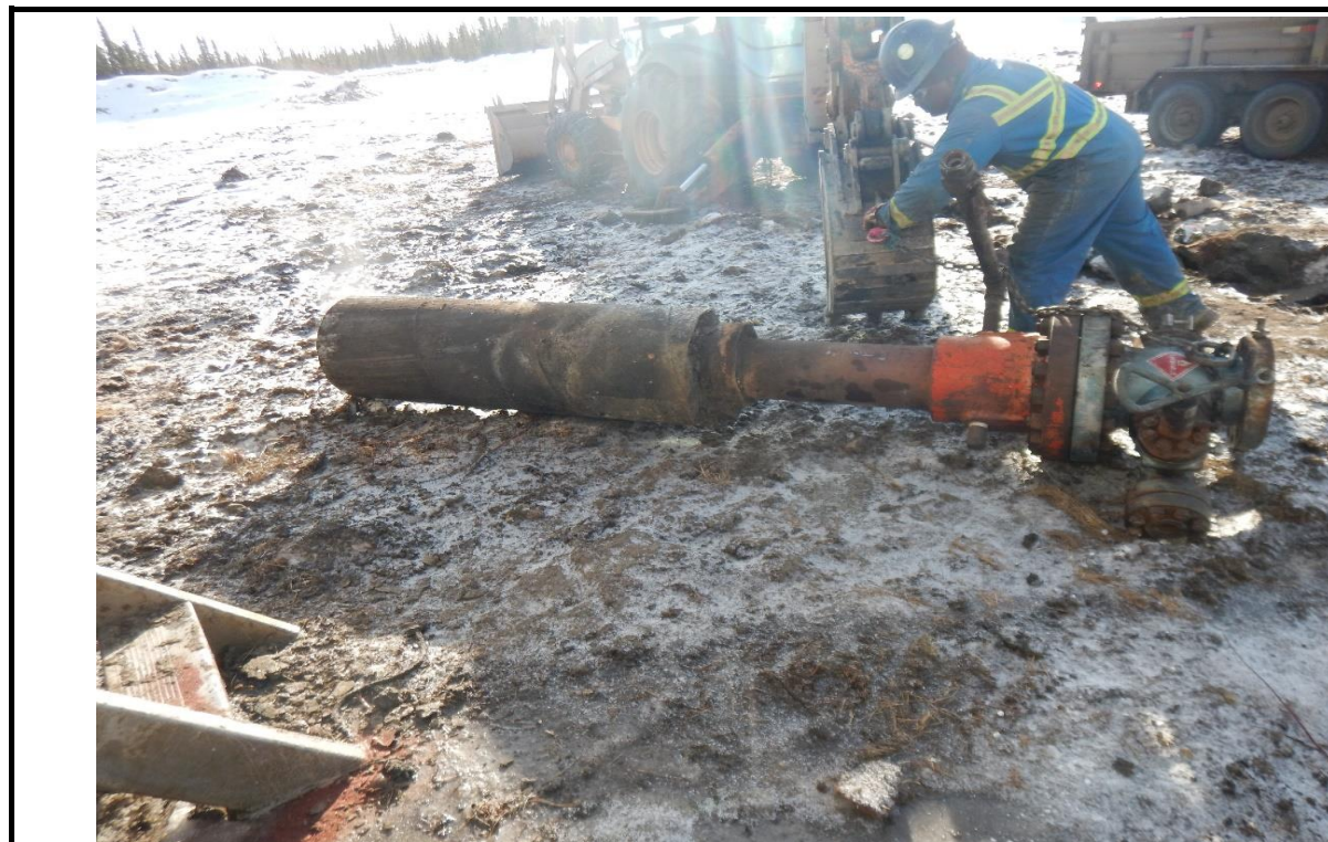
Wellhead pulled from ground
