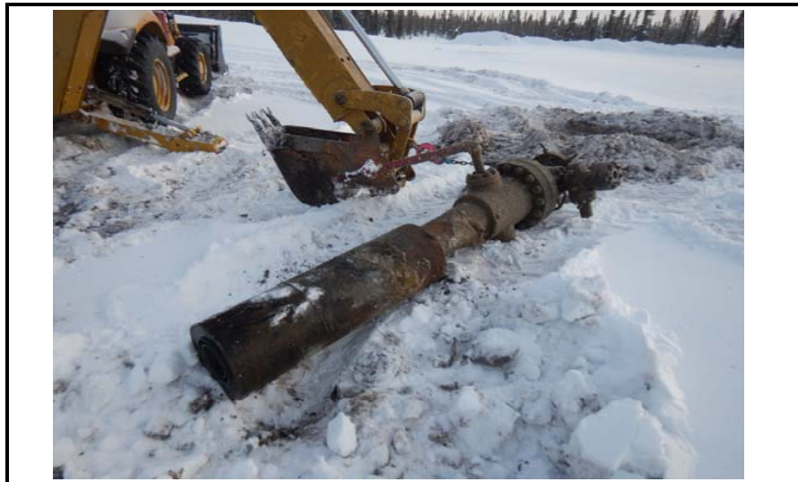
Wellhead removed from ground
