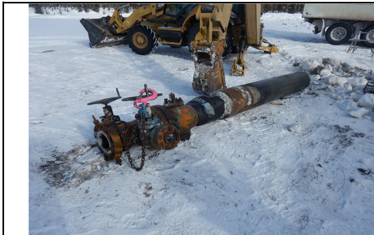
Wellhead removed from ground
