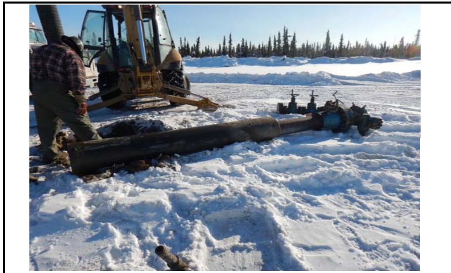
Wellhead cut off and pulled out of ground
