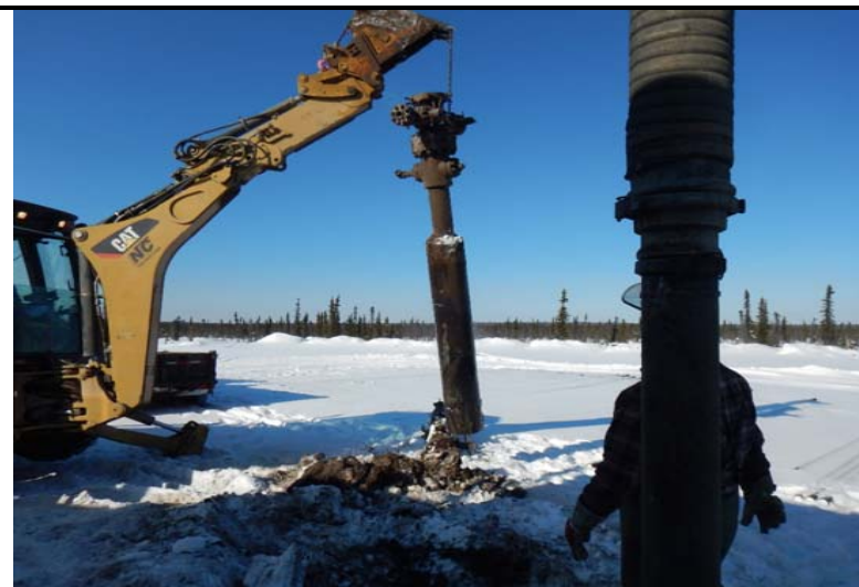
Wellhead pulled out of ground
