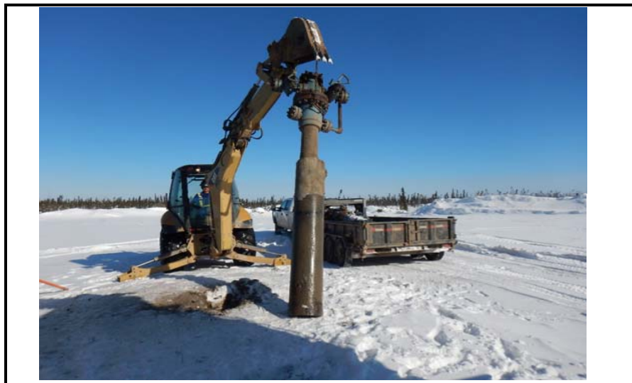
Wellhead pulled out of ground
