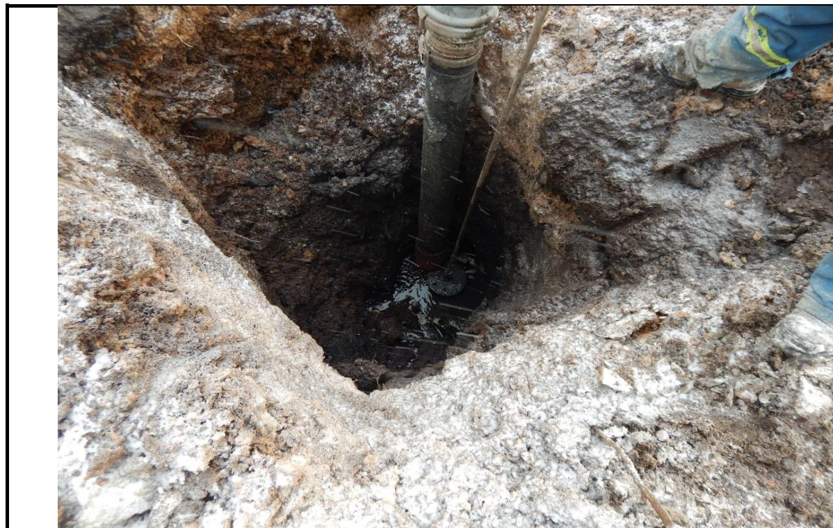
Vented cap installed into the casing
