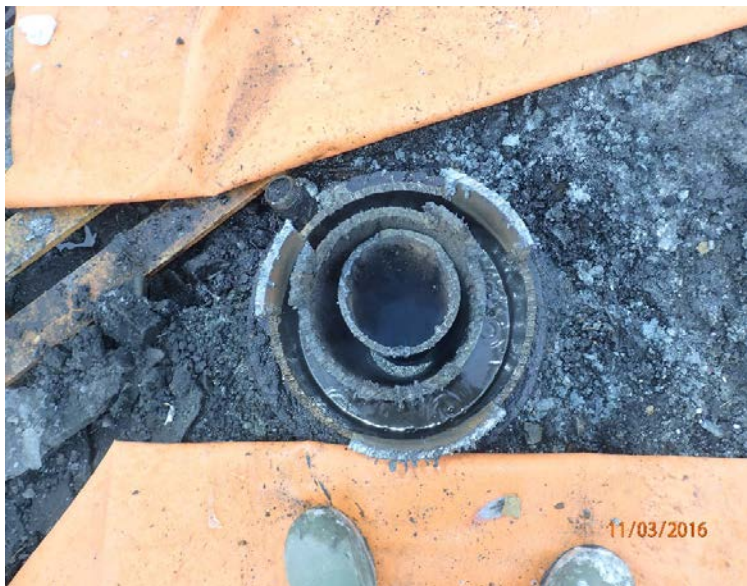
Casing string after wellhead off
