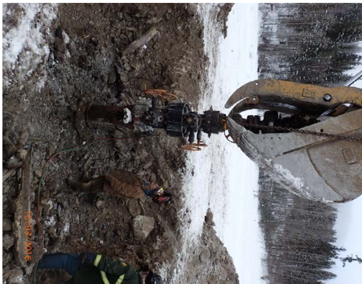
Hoe holding wellhead
