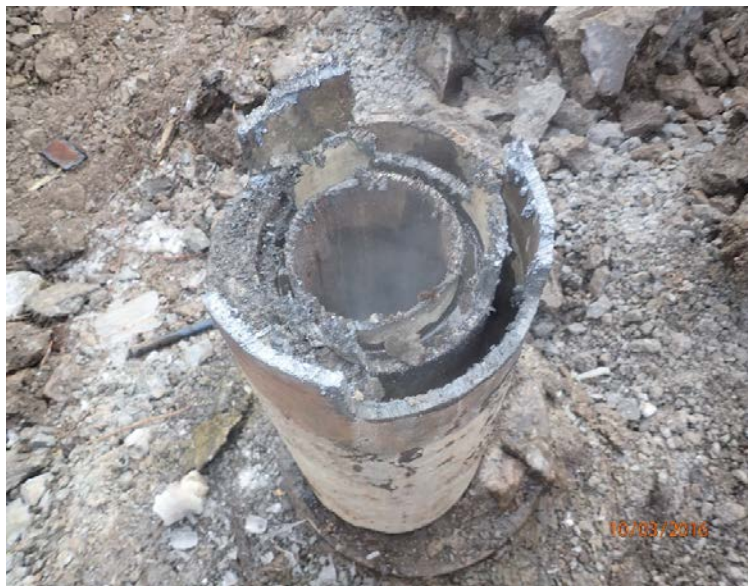
Cuts after wellhead off
