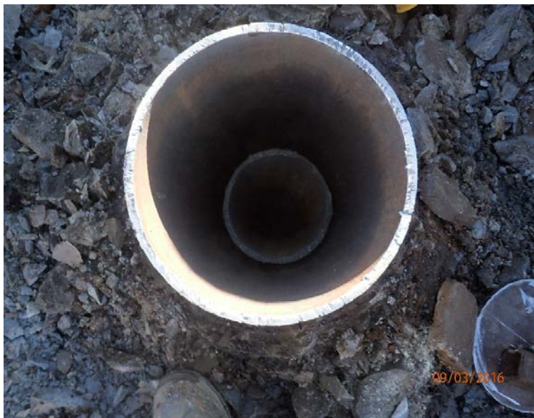
Casing strings after wellhead off
