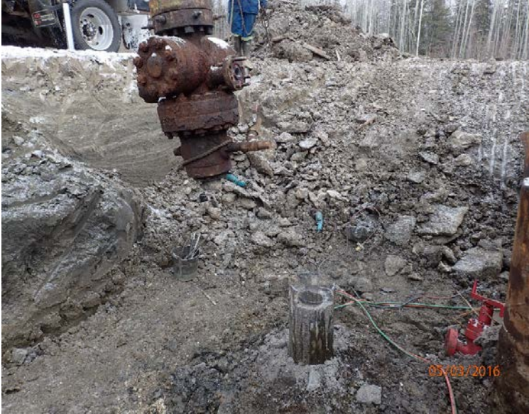
Wellhead being removed
