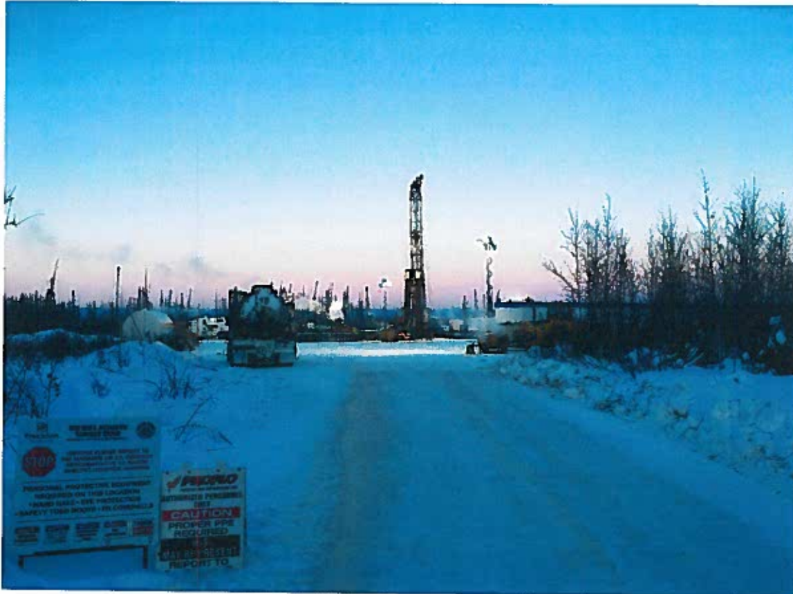
Photo#1: Hazard identification signs are present at the lease entrance.
