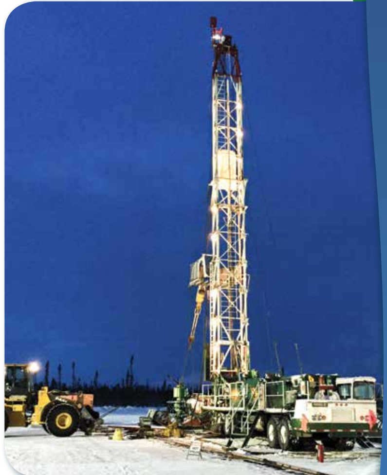
Service rig near Norman Wells, Northwest Territories, February 2016. (OROGO)
